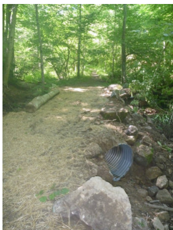
After repairs June 17th
