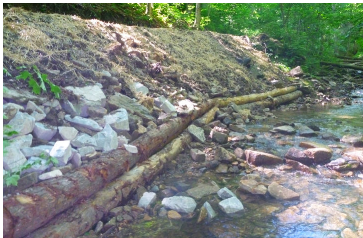
Mud Sill built June 15-16
